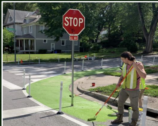
Quick build curb extension - Valentine and Wyoming
