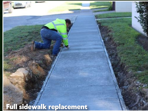
Full sidewalk replacement
