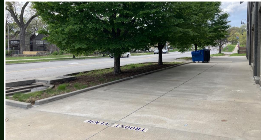
Curb extension rain gardens on Brush Creek Boulevard
